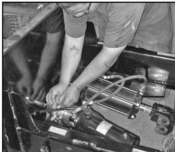
Figure 14. Attached to Support Structure.
