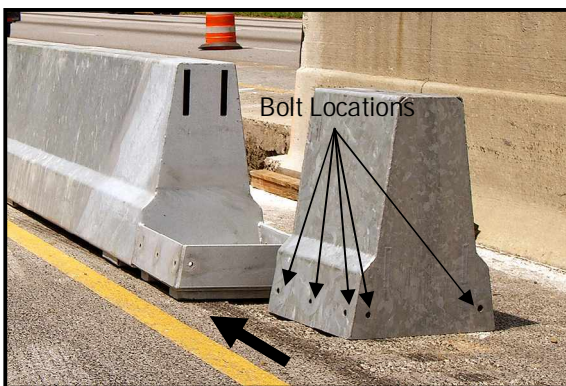
Figure 21. Slide the cover over the End Terminal. Attach the cover with the eight bolts around the base of the cover (both sides and end).
