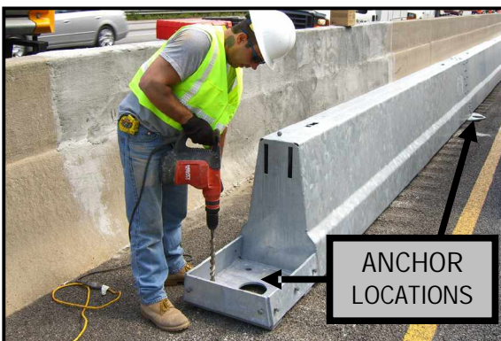
Figure 18. Drill the anchor bolt holes through the 4 holes in the end section.
