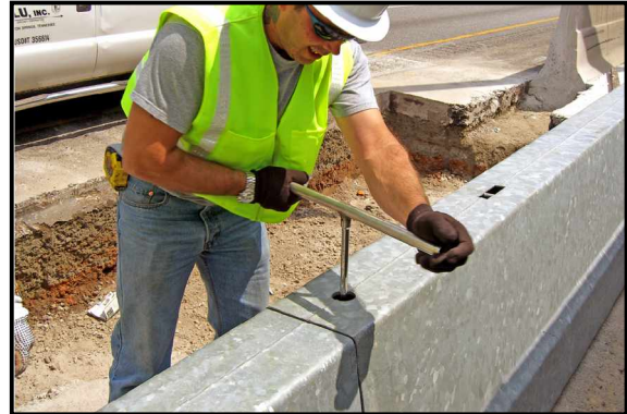
Figure 13. Tighten the retaining nut on top of the threaded stud
