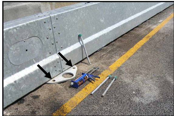
Figure 19. 6-meter anchor hole locations (concrete or Asphalt)
